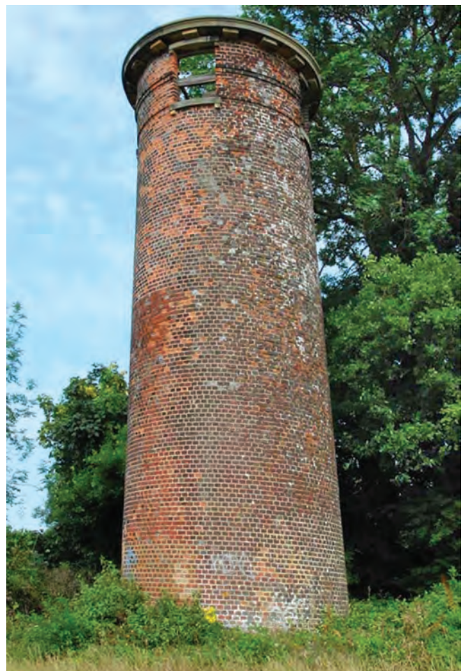
Merstham tunnel-surveying observatory tower
